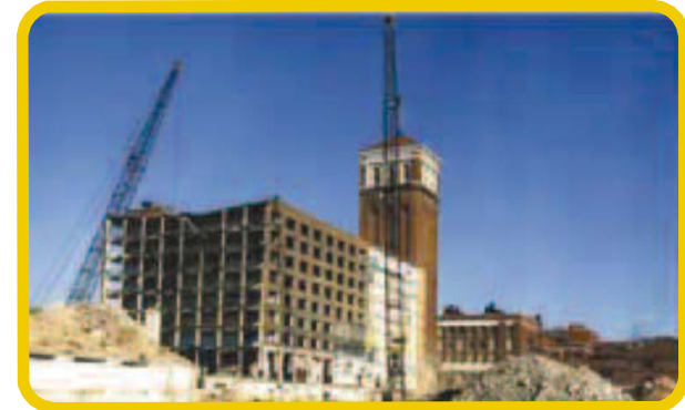
Sears Warehouse Construction Site
