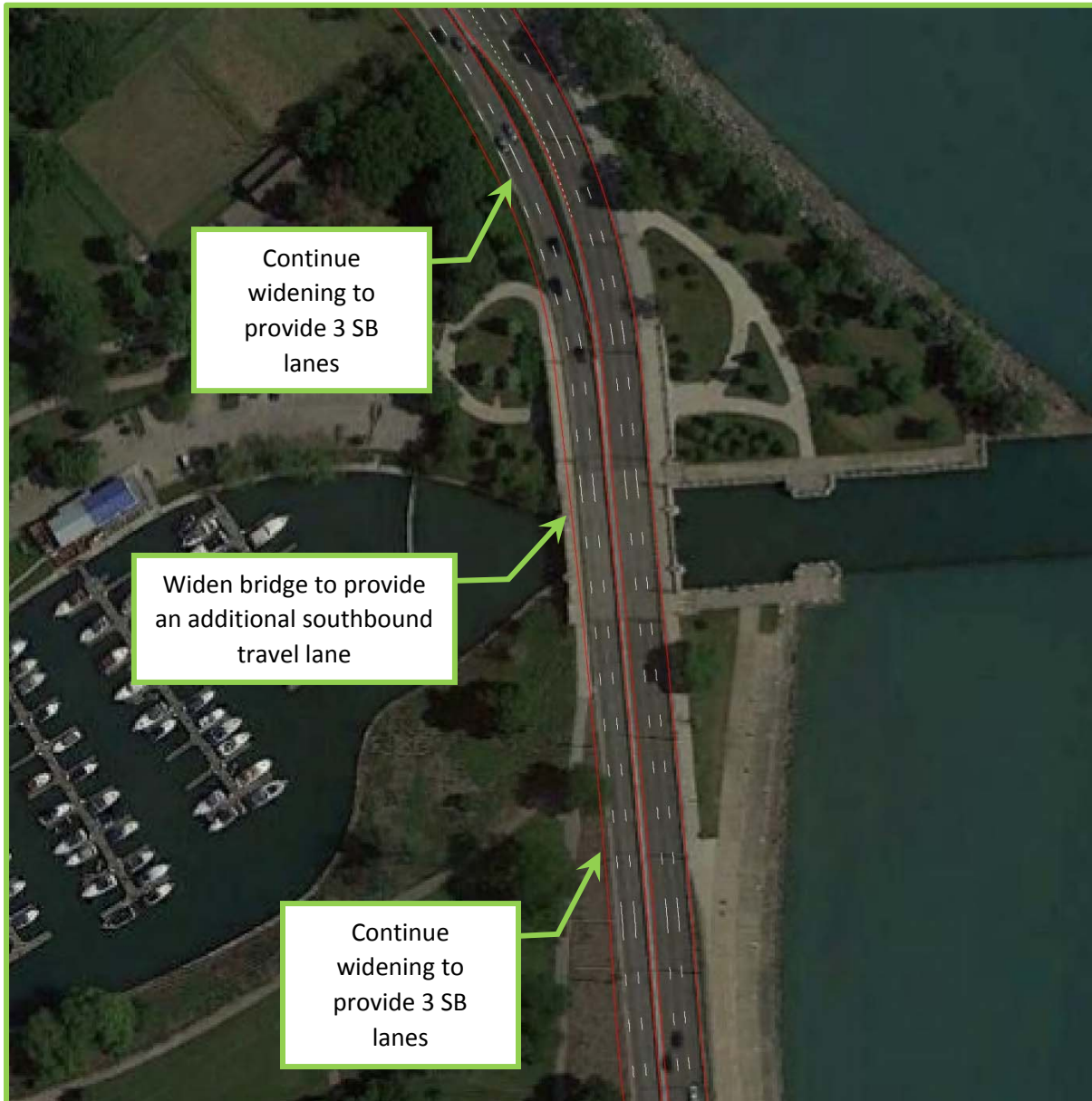
Figure 4-4: Lake Shore Drive at 59 th Street Harbor Bridge, Third SB Lane
