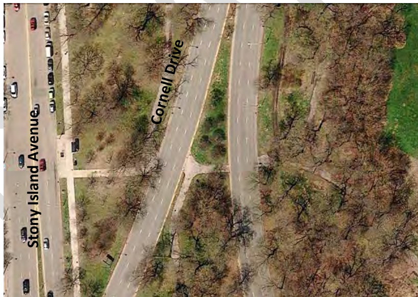
Unmarked Crossing of Cornell Drive near 65 th Street
