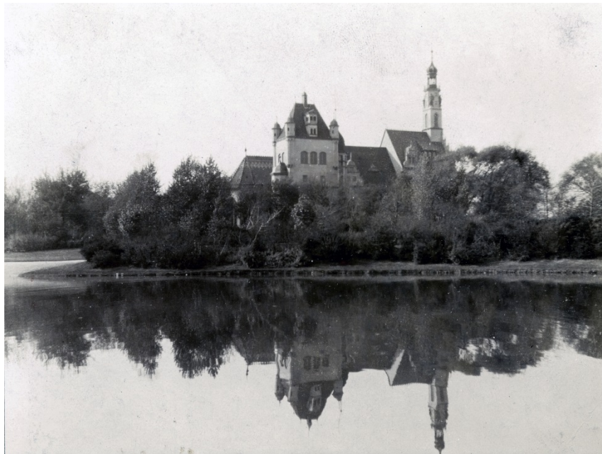
Photo 8: View of German Building looking northeast across 59th Street Inlet, 1904 (no longer extant), Regenstein Library, University of Chicago LNE-UC-04510-1904
