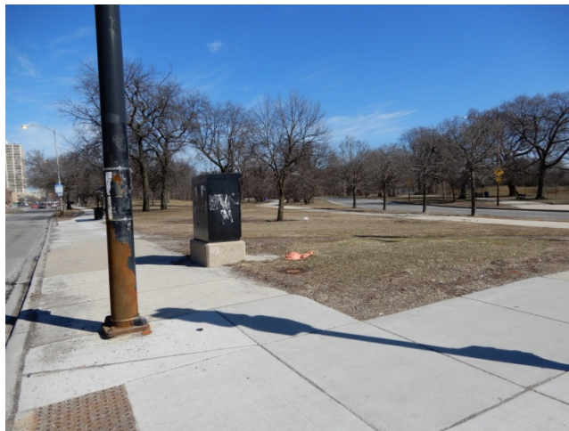
Photo 24: Flat topography at Western Perimeter's southwest corner at E. 67th and S. Stony Island Avenue. View looking northeast with S. Stony Island Avenue on left, S. Cornell Drive and subtle berms in distance
