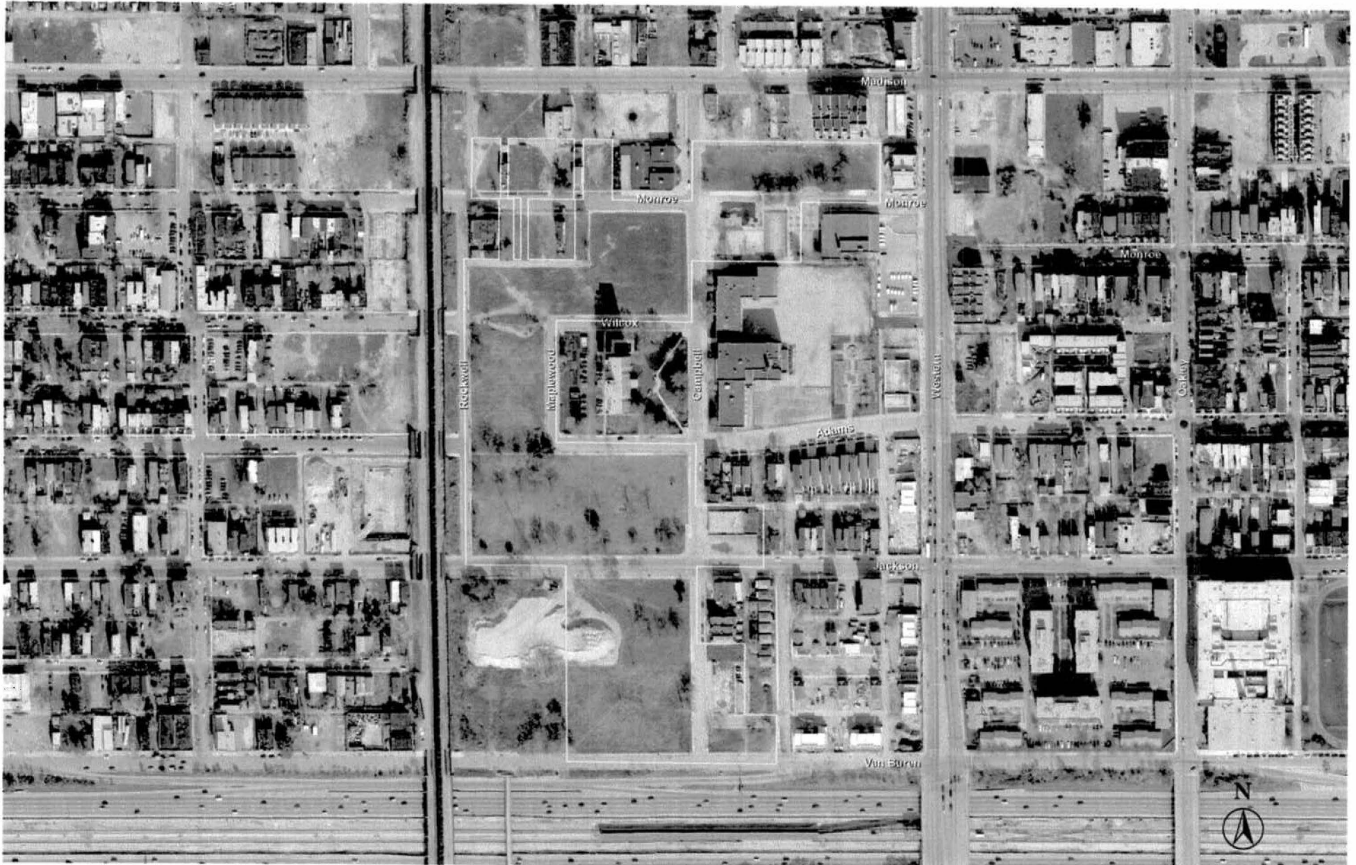
Rockwell Gardens Hope VI Redevelopment Chicago Housing Authority
