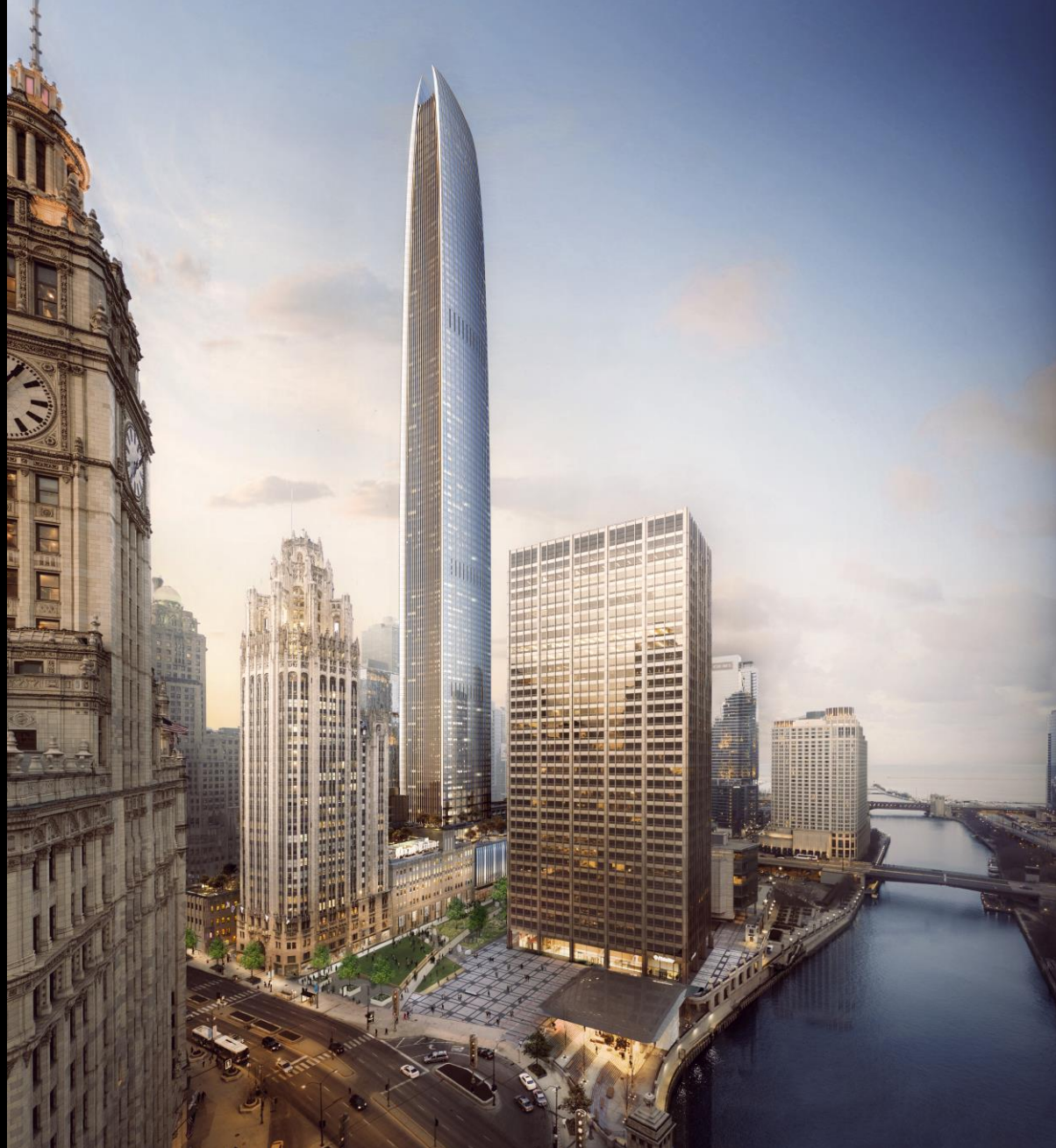
AERIAL VIEW FROM SOUTHWEST DIRECTION
