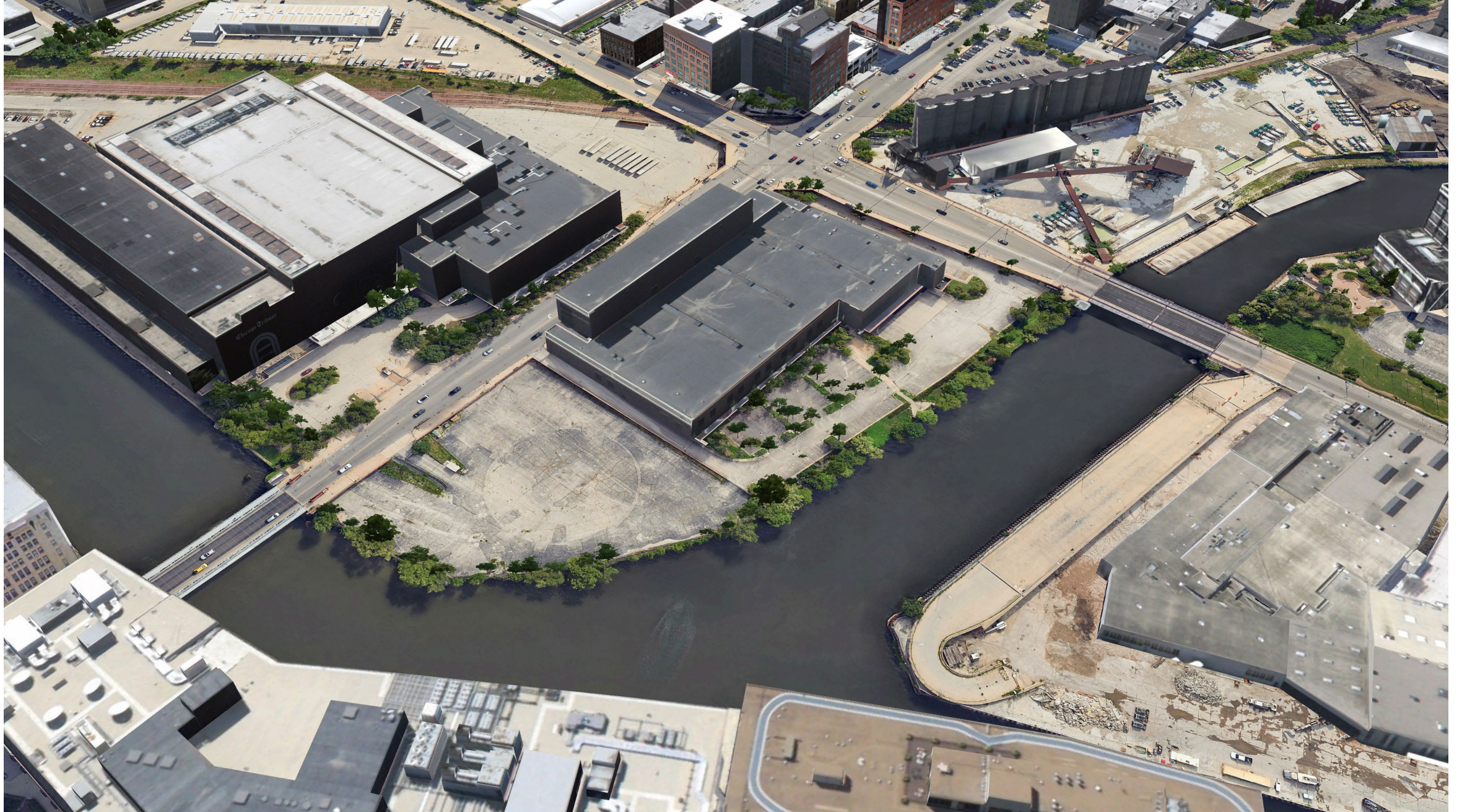
EXISTING AERIAL VIEW FROM NORTHEAST
