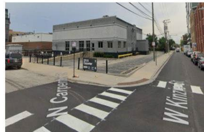
EXISTING CONDITIONS ALONG KINZIE
