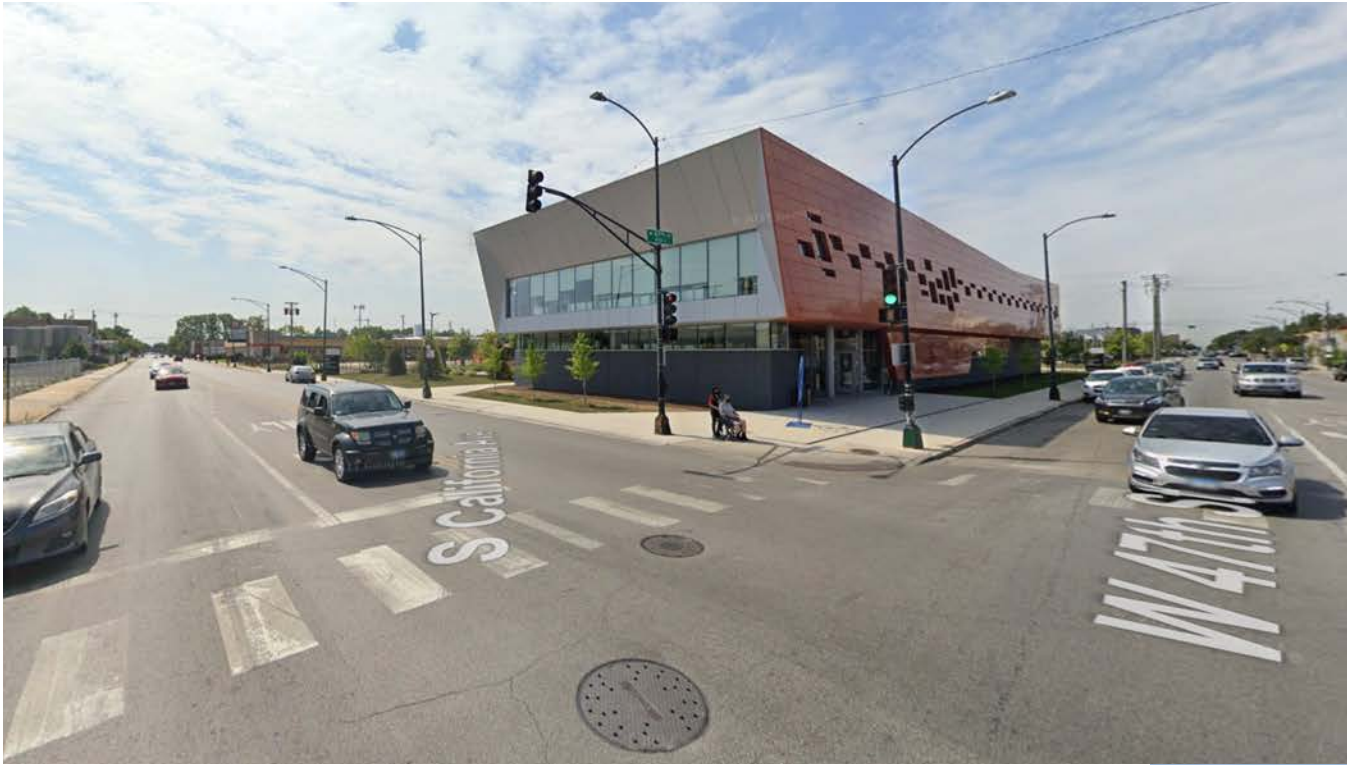
View of existing facility, looking southwest
