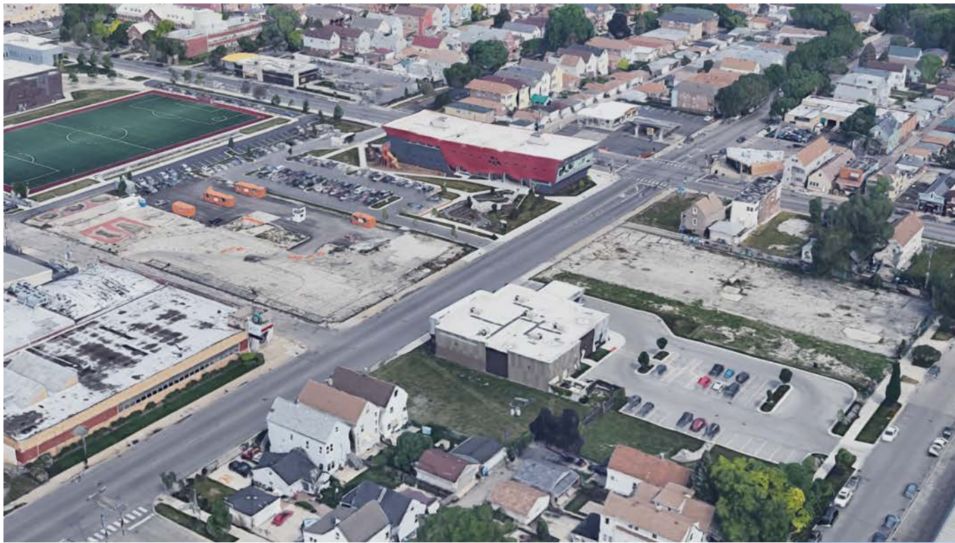
Aerial view of project site, looking northwest
