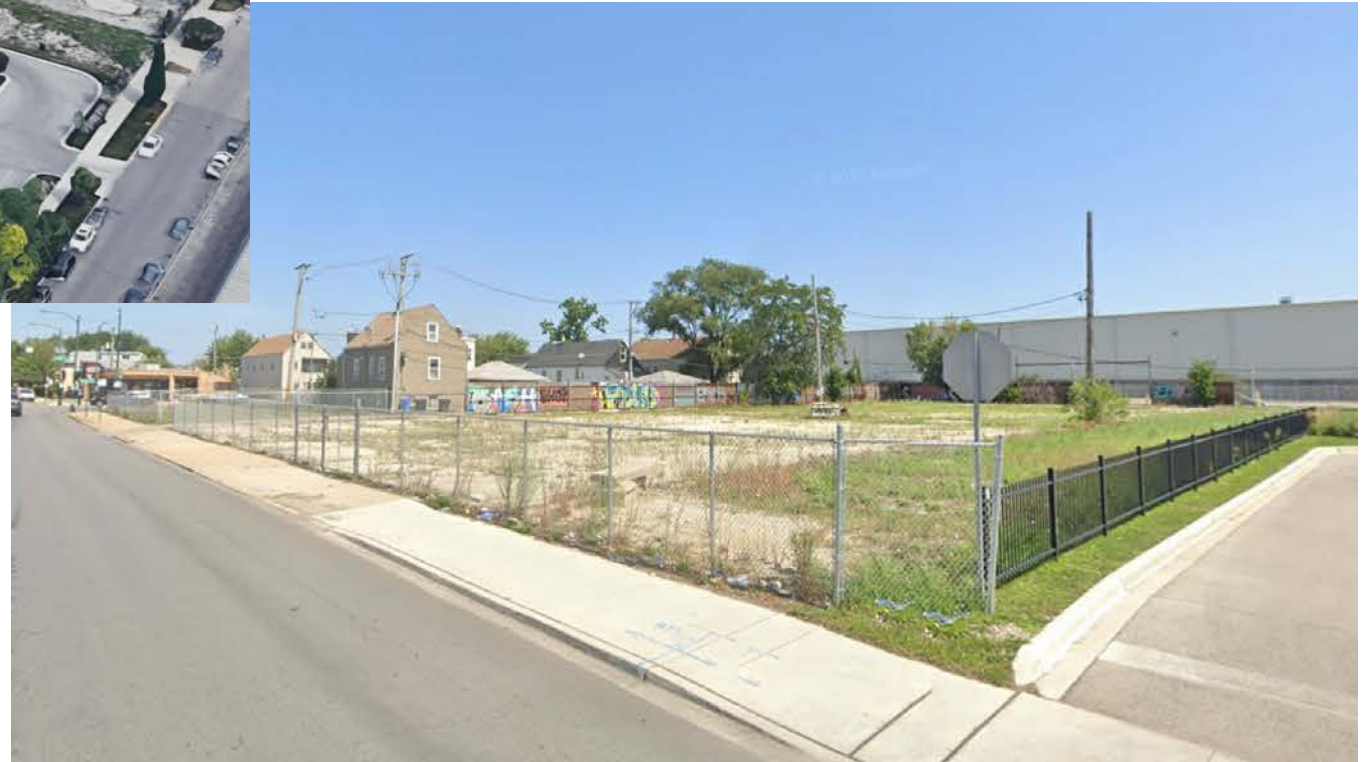
Site of new parking, looking northeast
