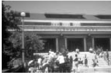
Community facility at Eckhart Park
