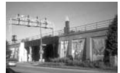
The Union Pacific Viaduct along Hubbard Street
