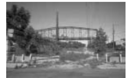
Vacant property along the Union Pacific Viaduct near Kinzie Street
