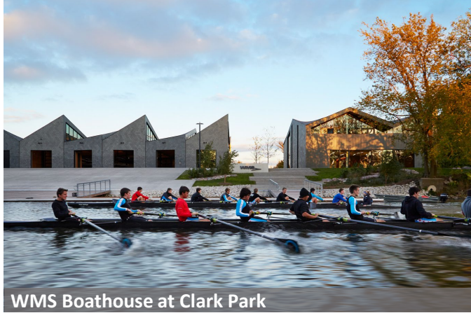
WMS Boathouse at Clark Park
